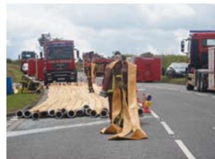
The High Volume Pump in action
